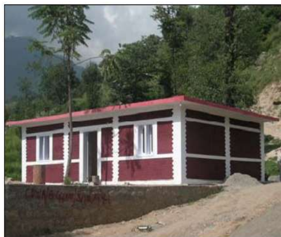
Fig 15: Finished confined masonry structure showing seismic reinforcement
