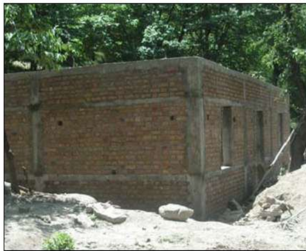
Fig 14: Under construction confined masonry structure
