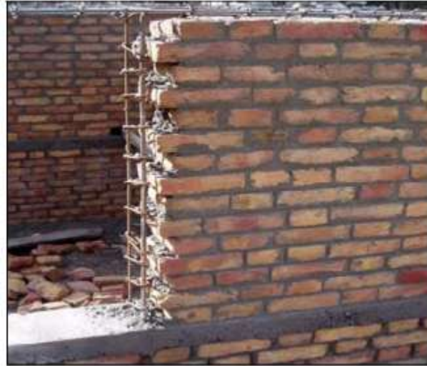
Fig 13: Vertical reinforcements around openings
